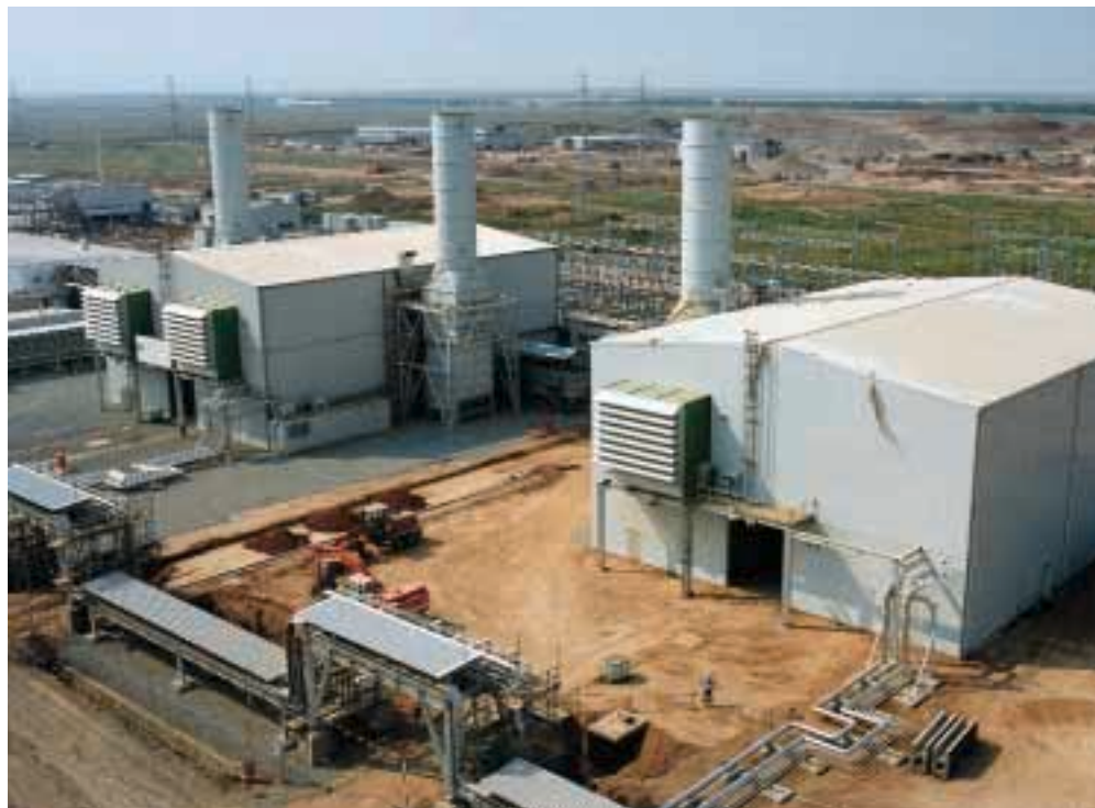
Complete... the power station units at KPC
