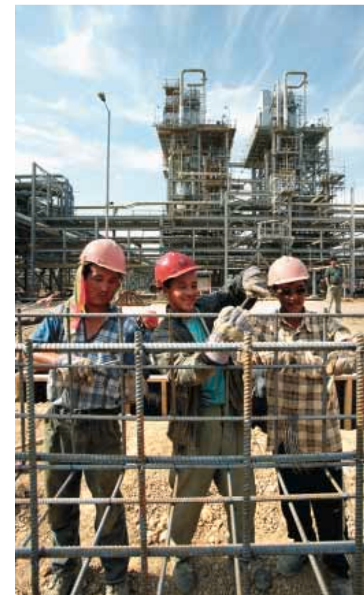
Work at Unit 2, August 2002
