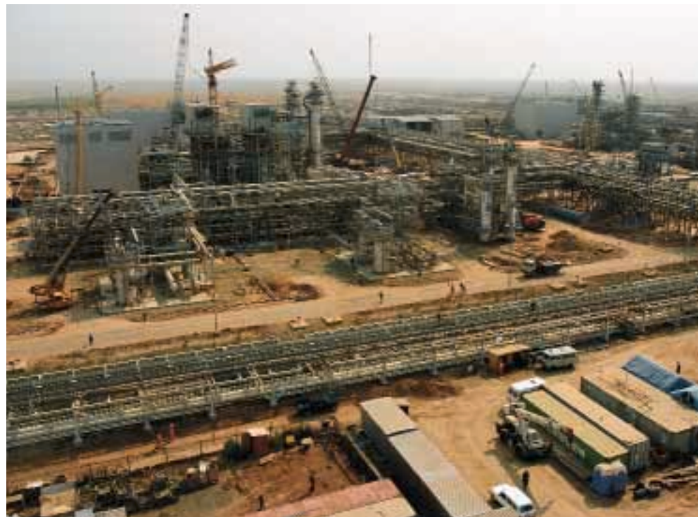
KPC under construction in August, 2002
