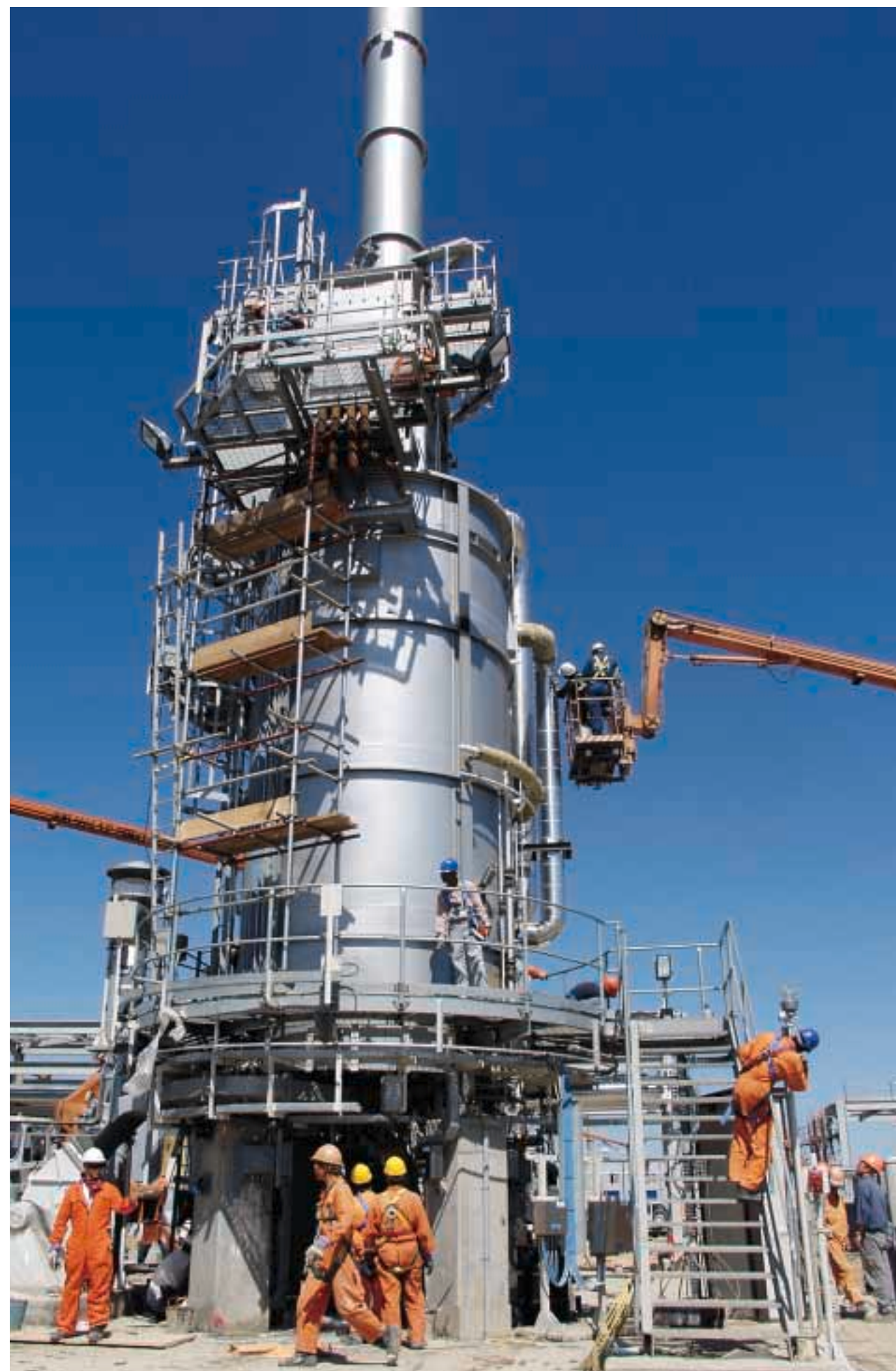
The hot oil system is completed
